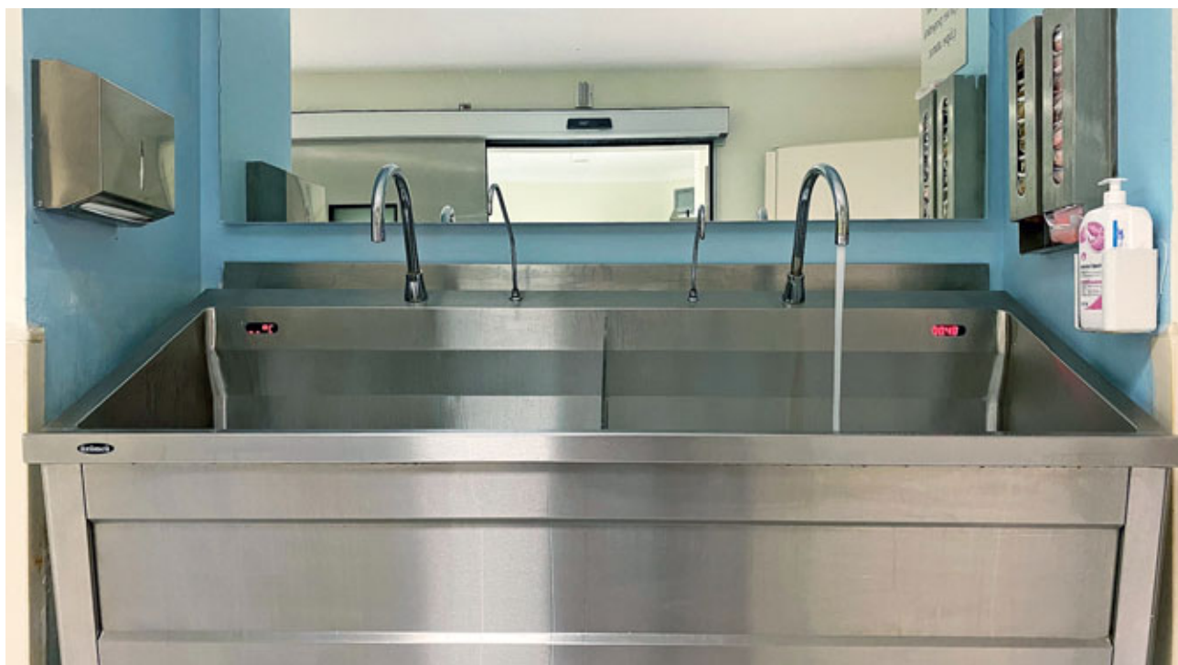
Fig. 1. Standard sensory taps are designed for operating theatre.
